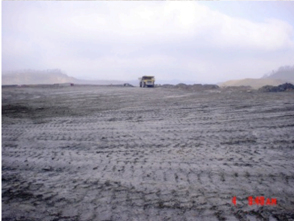
Figure 4. Surface mines partway through the reclamation process. By use of heavy machinery, the ground is highly compacted (above). While this temporarily improves land stability, it is not a conducive medium for plant growth, especially native tree growth (below).
